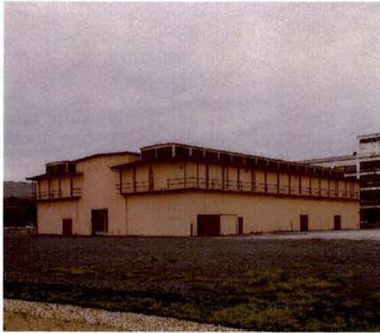
1 BUILDING 173 - LUMBER STORAGE SHED, BUILT 1918-1919
