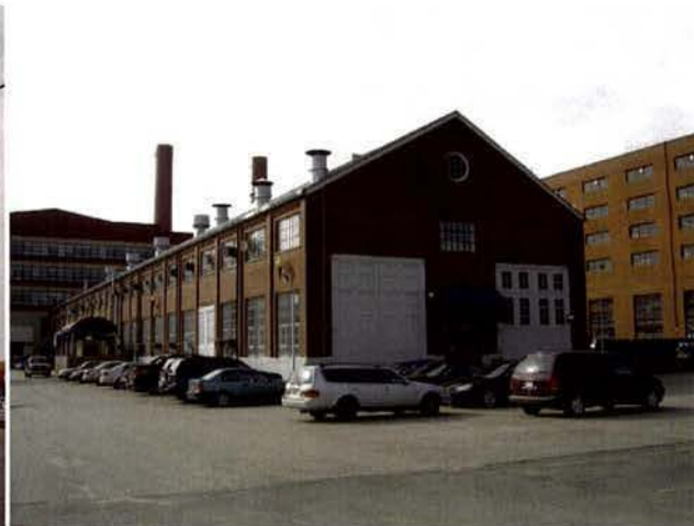
6 BUILDING 74 - TRANSPORTATION REPAIR SHOP, BUILT 1938
