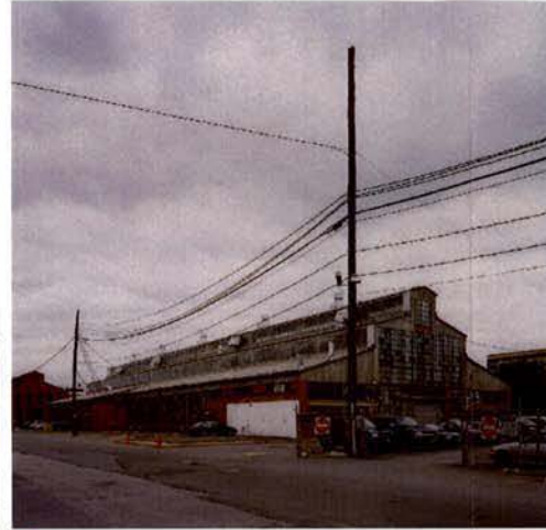
3 BUILDING 167 - BOILERMAKER'S SHOP, BUILT 1919
