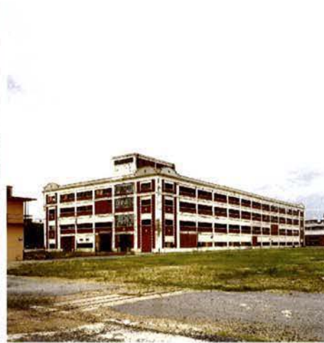
2 BUILDING 160 - PATTERN & JOINER SHOP, BUILT 1917
